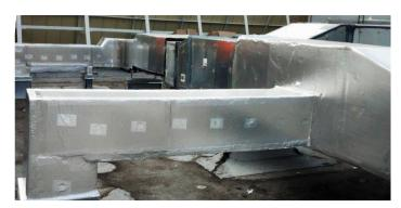
**PRO TIP:** To cover washers, cut out squares of jacketing at approx 6". Adhere the patches over the washers. Squeegee in place.
