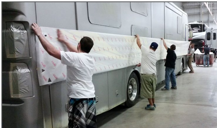
Lightweight papers are commonly used for the installation of RV spray.
